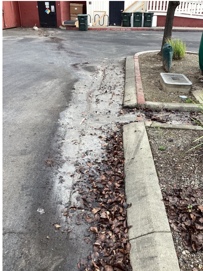
Apparent private sanitary sewer overflow originating from the Lucille's cleanout and draining to the storm drain inlet.
