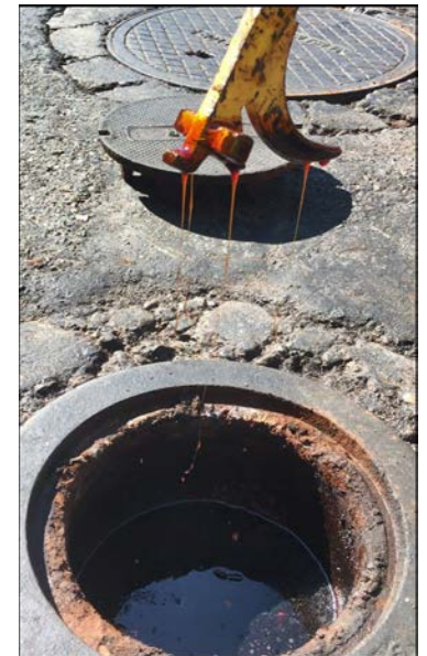
Grease accumulation downstream of Lucille's – CCTV on February 13, 2023
