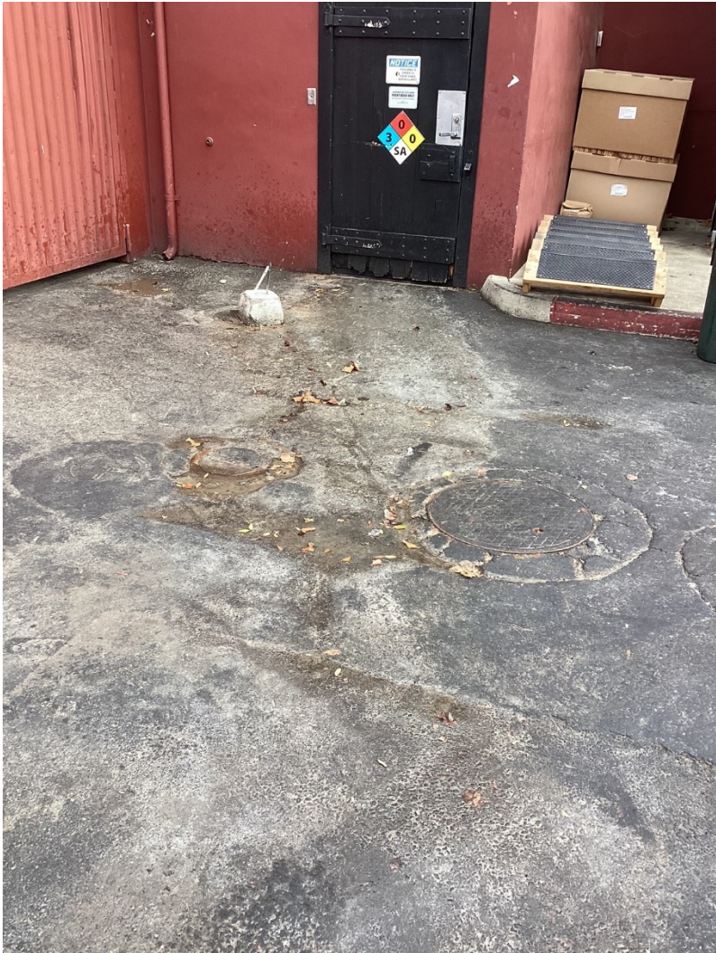
Apparent private sanitary sewer overflow originating from the Lucille's cleanout and draining to the storm drain inlet.
