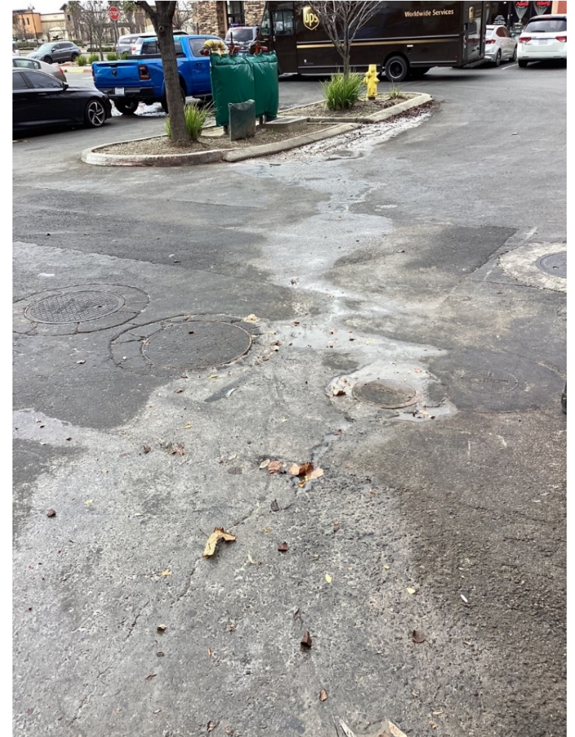
Apparent private sanitary sewer overflow originating from the Lucille's cleanout and draining to the storm drain inlet.
