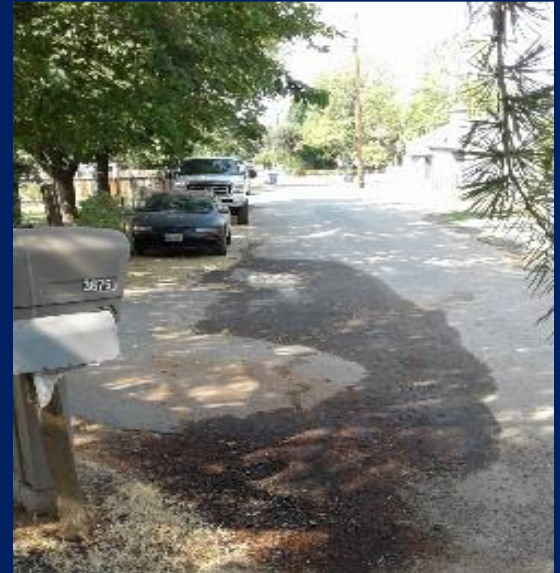
Overflow from clean out
