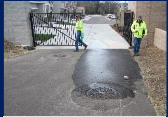
Manhole overflowing
