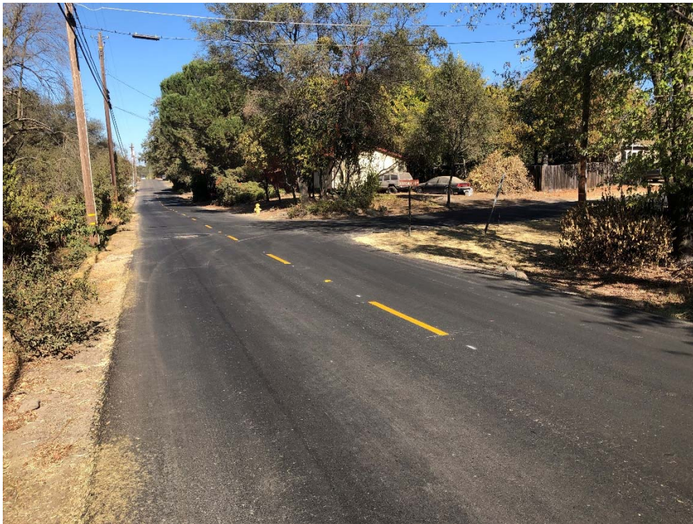
Looking north on Aguilar Road.
