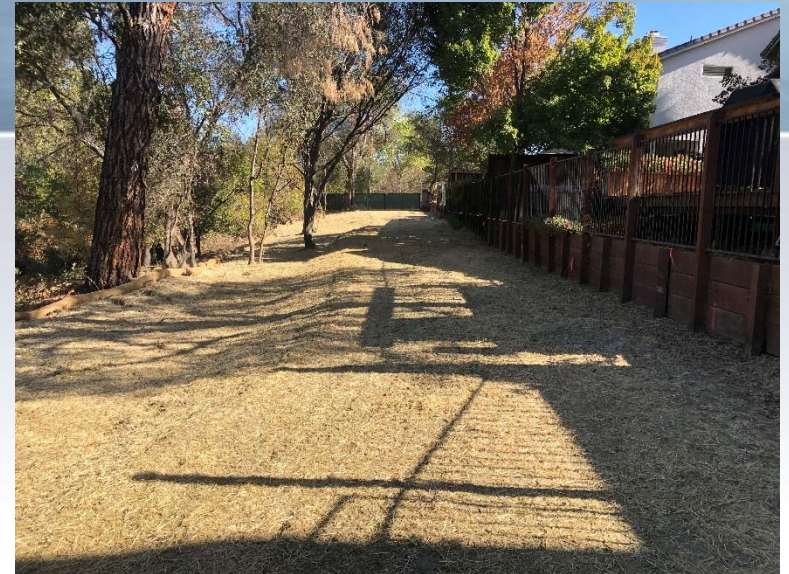
GrassPave2 access road behind Corona Circle.
